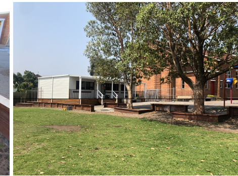
(M) DRY CREEK TO EDGE OF FIELD. WITH POTENTIAL FOR WATER BY INTRODUCTION OF TAP (UTILISING BORE WATER ON SITE IF WATER QUALITY APPROPRIATE) SITE VERY FLAT SO MAY NEED TO EXPLORE DRAIN / PLUGS.
